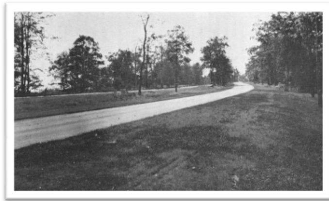
Demonstration Mile southbound in vicinity of Overlook Palisades Interstate Parkway
