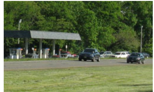
Existing northbound gas station along the Palisades Interstate Parkway. Note how the galvanized light fixtures show prominently against the landscape.
