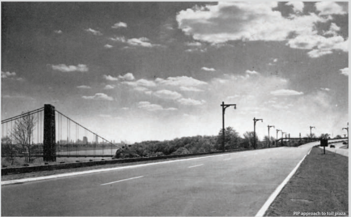
PIP approach to toll plaza
