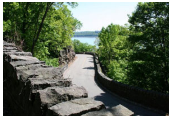
Photo of Henry Hudson Drive hairpin curve showing parapet walls Photo Courtesy of Paul Daniel Marriott
