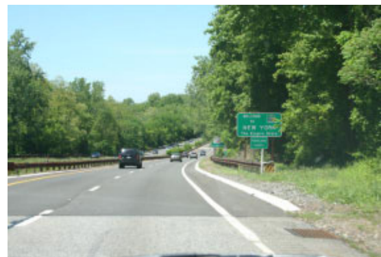
Photo of the Palisades Interstate Parkway showing no curb in the New Jersey section and a white curb in the New York section
