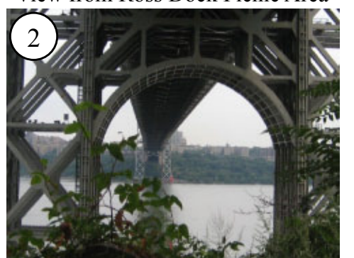
View of the GW Bridge from HHD
