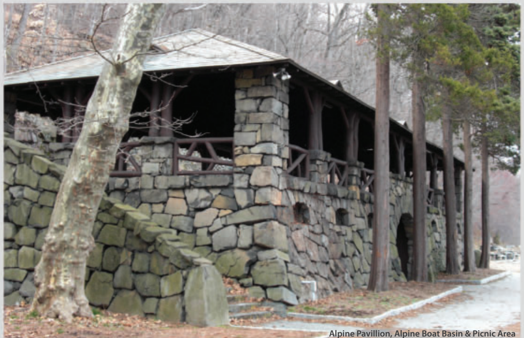
Alpine Pavilion, Alpine Boat Basin & Picnic Area
