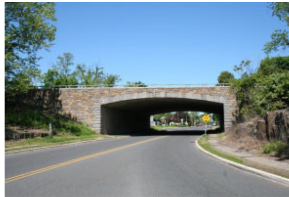
A current photo of the same bridge Photo Courtesy of Paul Daniel Marriott
