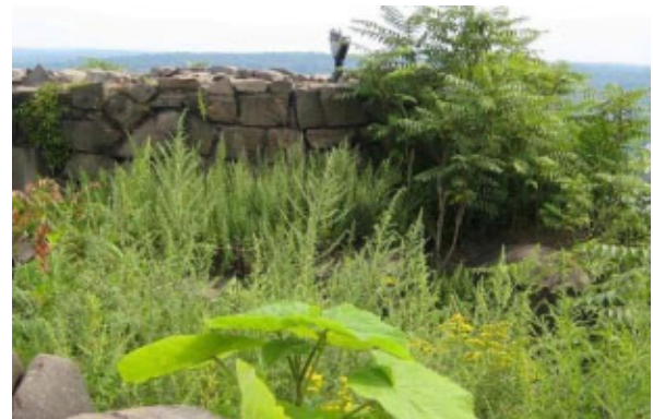
Weeds and invasives have become overgrown and obstruct views at Lookouts
