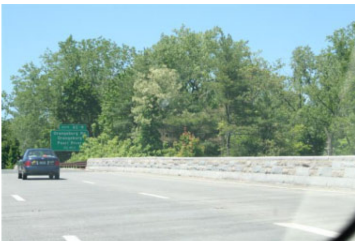
Parapet wall in New York State
