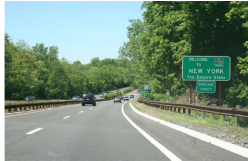
The gateway signage was removed from the median and MUTCD compliant "Welcome to New York and New Jersey signs were added.
