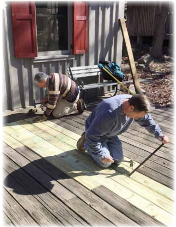
Repairing the Visitor Center deck
